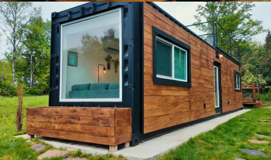
40 ft refurbished container converted into a one-bedroom open-plan home, with flexibility to be adapted into a two-bedroom layout.
